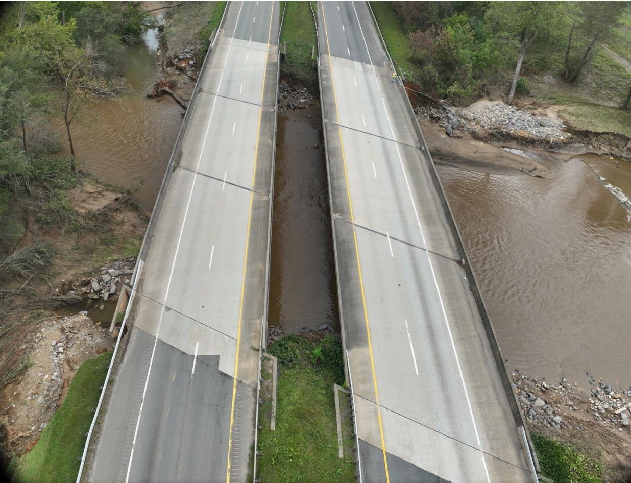
UAS team on TSMO Unit mission discovers compromised bridge with massive scouring, still fully open to traffic
